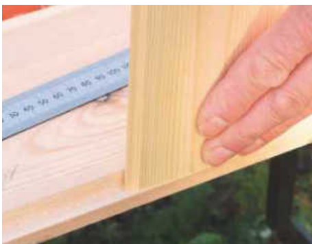
STEP 8. Check the matchboard is a snug fit in the rebates. This will be neater if slightly inset
